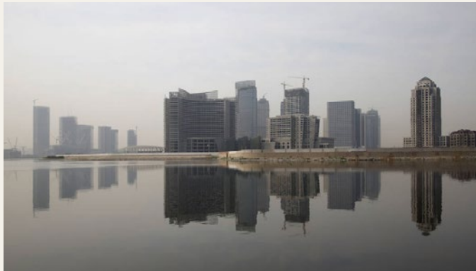
Unfinished construction in China's "Manhattan of the East," located in Yujiapu (于家堡金融區), Tianjin.
