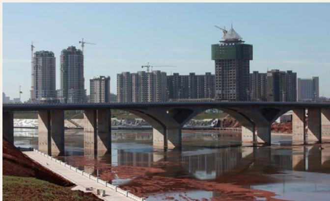
Abandoned partially-constructed buildings in Kangbashi, Inner Mongolia, China's most-famous ghost city.
